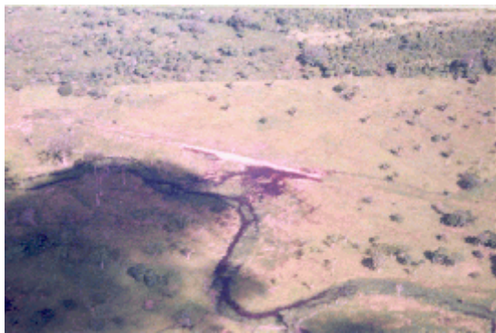
OIL SPILL: An attack on the Cano-Limon pipeline results in oil runoff into a nearby stream. Although the pipeline is several feet underground (located at center, running diagonally), Arauca's flat terrain makes it an easy target for terrorists.
